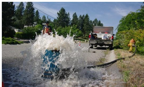
Flushing in Progress
